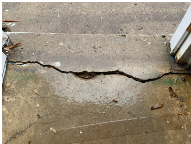
Crack in doorway
