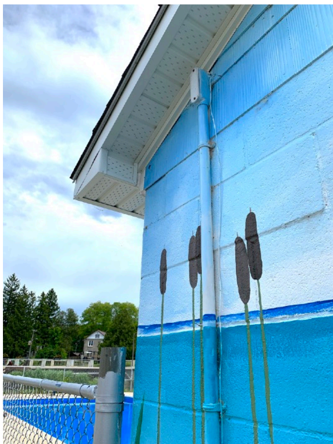
New vented soffits and fascia installed
