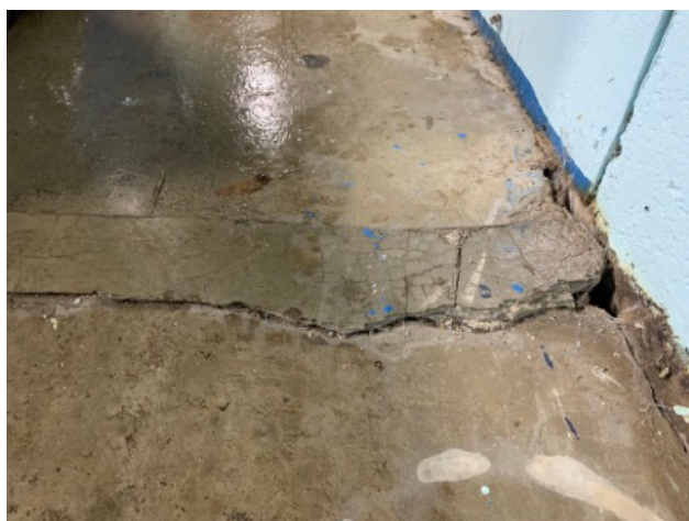
Large crack in main entrance
