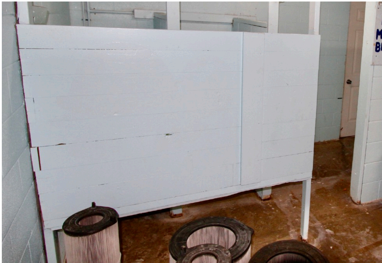
Boys toilet area divider rotten at floor and blocks cleaning
