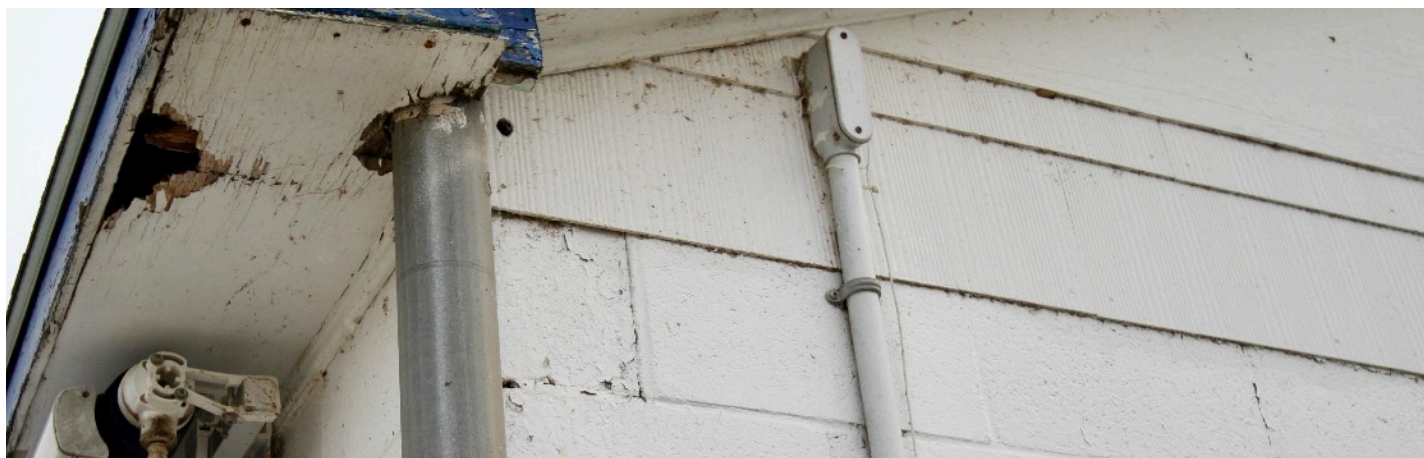
Existing Soffits - Rot and no vents.
