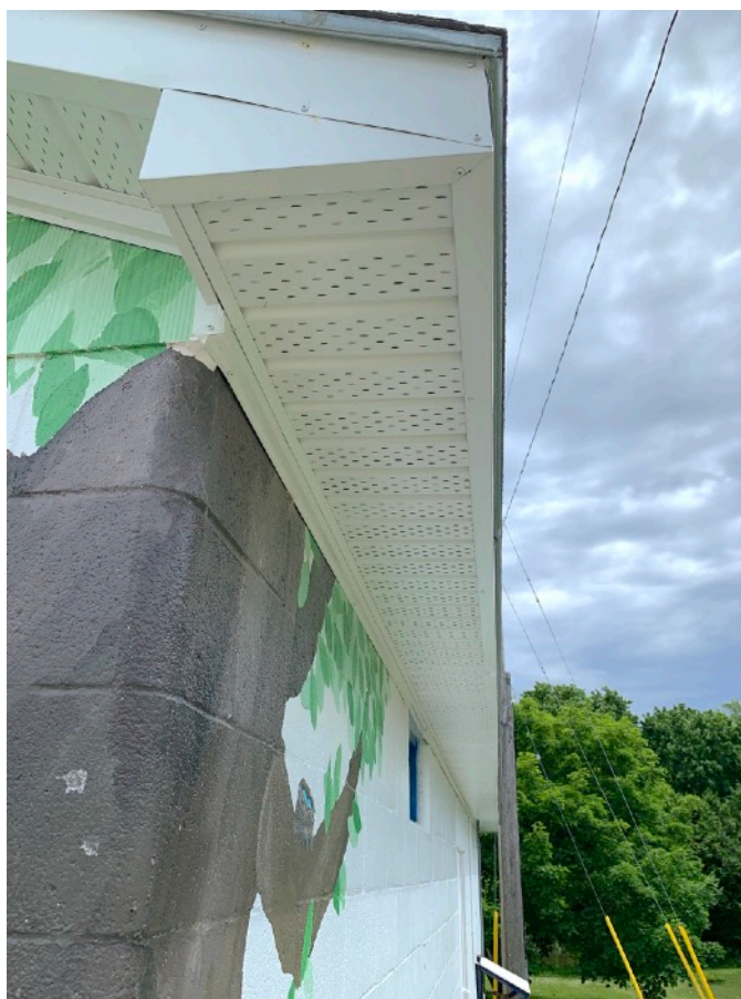
New vented soffits and fascia installed
