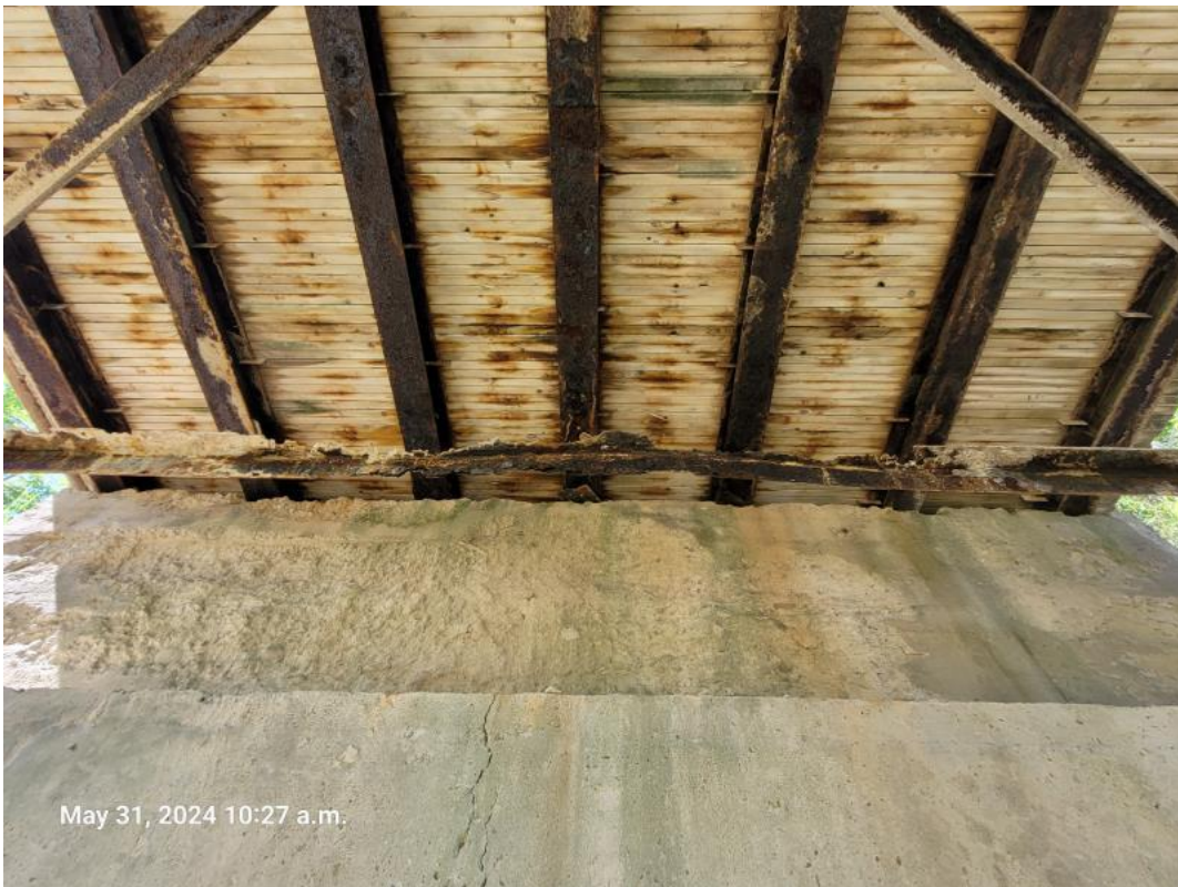
4-South Abutment and South Stringer
