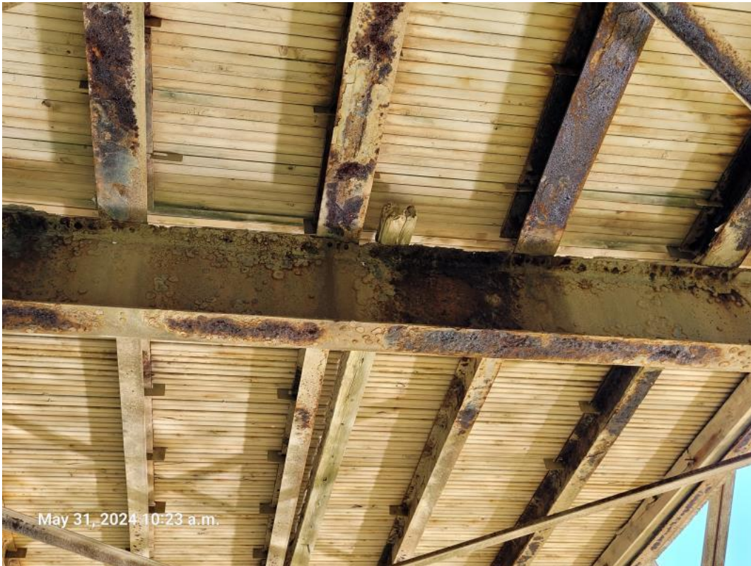
3-Soffit Looking North
