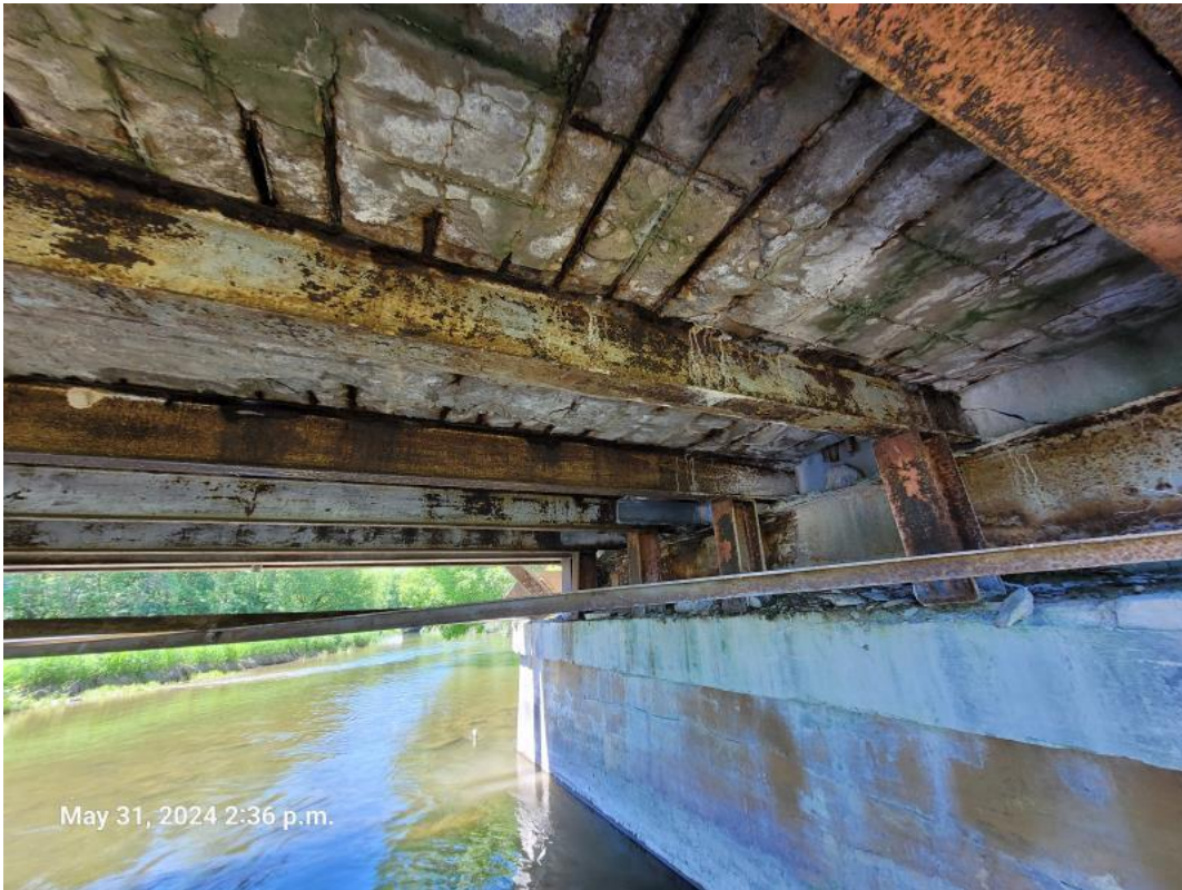
5-Soffit and Stringers at North End (1)
