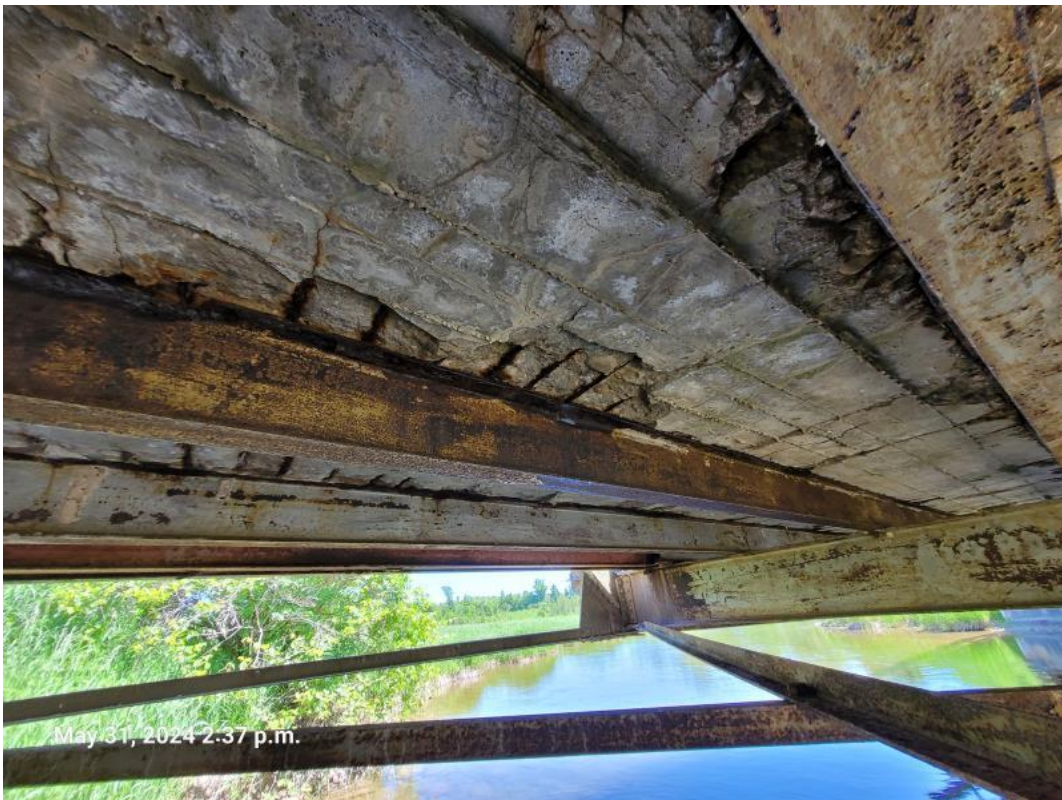
6-Soffit and Stringers at North End (2)
