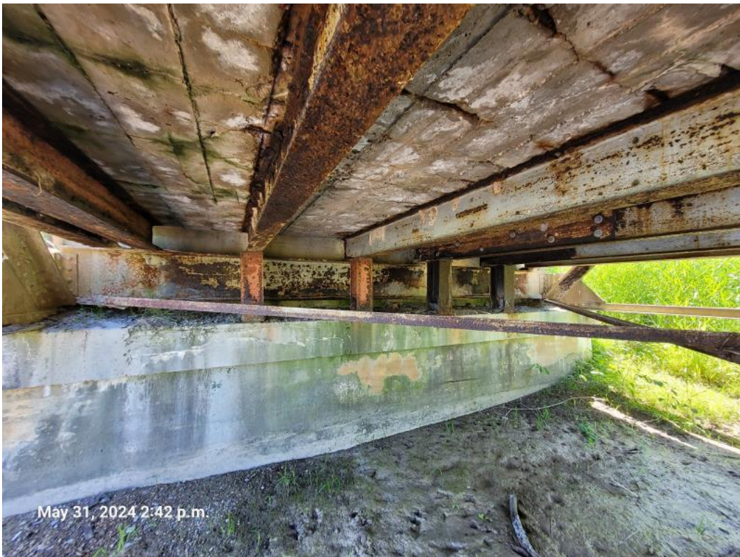
4-Soffit and South Abutment
