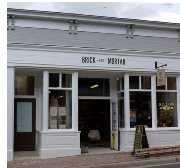
Painted brick, base and transom, and cornice detailing
