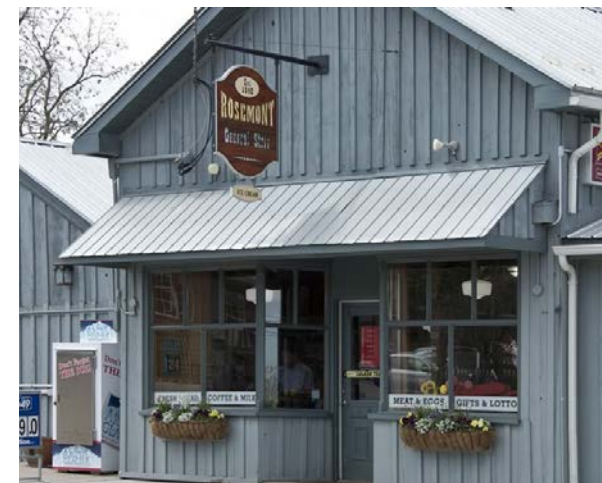
Board and batten exterior
