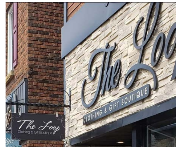
Stone veneer facade
