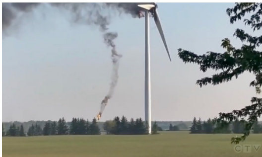
Fig. 1 Typical wind turbine fire (Kingsbridge 1 2024-06)
