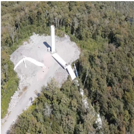
Fig. 2 Typical tower collapse (Bow Lake 2021-08)
